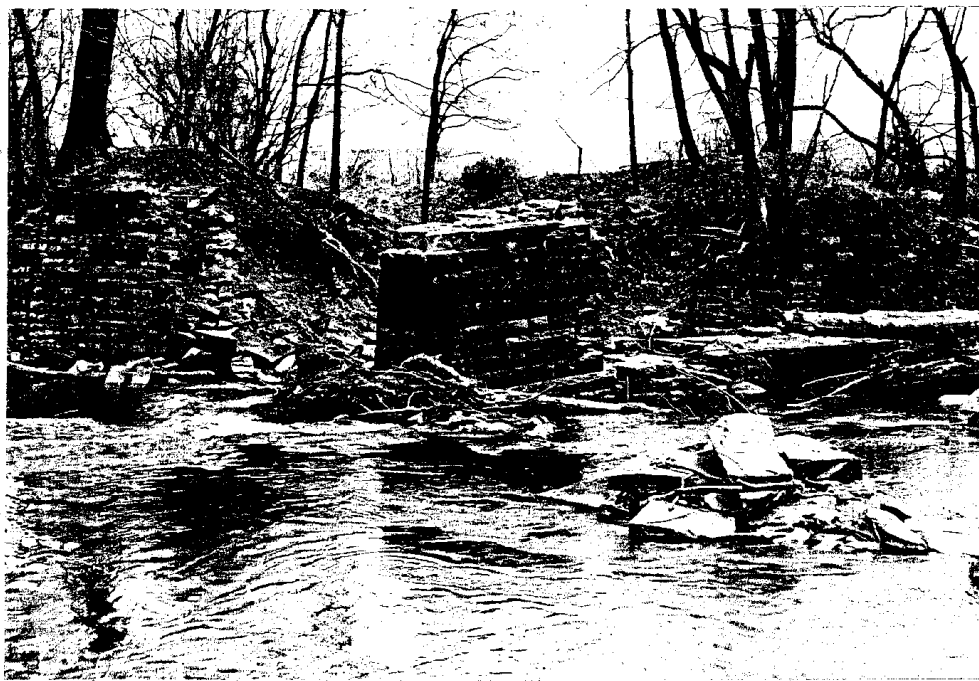
Figure 48. Ruins of the Briar Creek aqueduct, 800 feet south of U.S. Route 11 in Briar Creek borough, Columbia County. Most of the stone blocks are Keyser-Tonoloway limestone.
