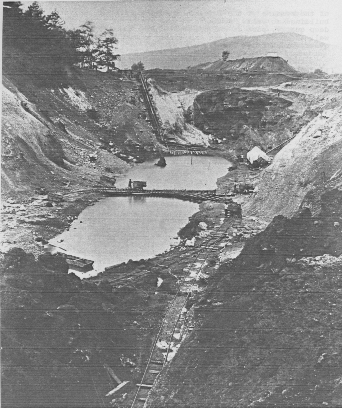
Figure 10. The iron ore pit at Pine Grove Furnace in about 1875. The pit is now Fuller Lake. Photograph courtesy of the Cumberland County Historical Society.
