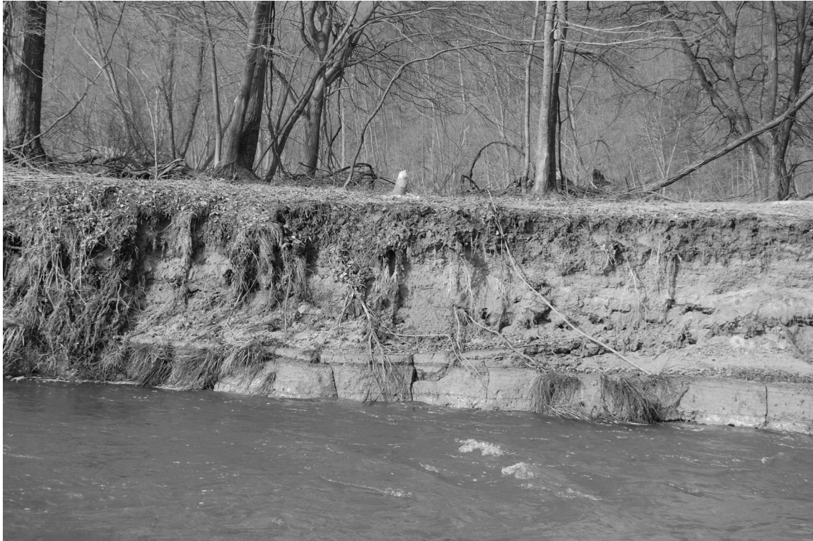
Figure 25. Legacy sediments at profile at STOP E. Rebars are beneath small orange flag. Photo 3/7/08 shortly after flood of 3/5.
