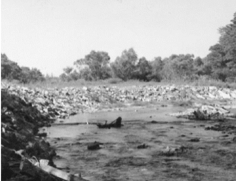
Figure 18. By 6/26/1987 rip-rap had apparently been added to the west side of the channel. PA DEP Photo.
