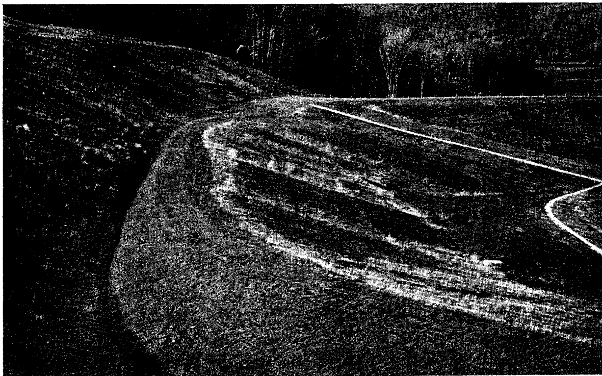
A. Part of the surface drainage configuration at the repaired toe of the Tioga landslide. The right (east) abutment of the Tioga Dam is in the background.
