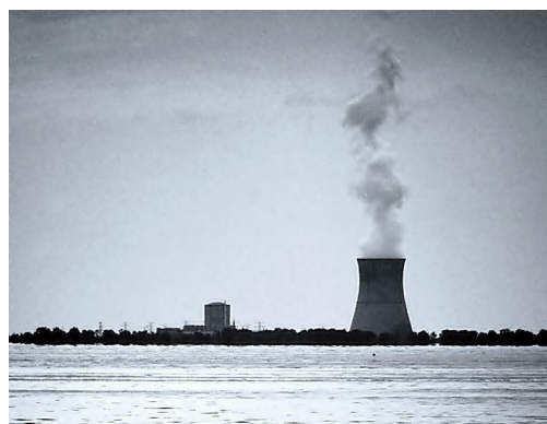
POI Figure Source: Davis Besse Power Plant, n.d., https://commons.wikimedia.org/wiki/File:Davis_besse_power_plant-CN.jpg .
