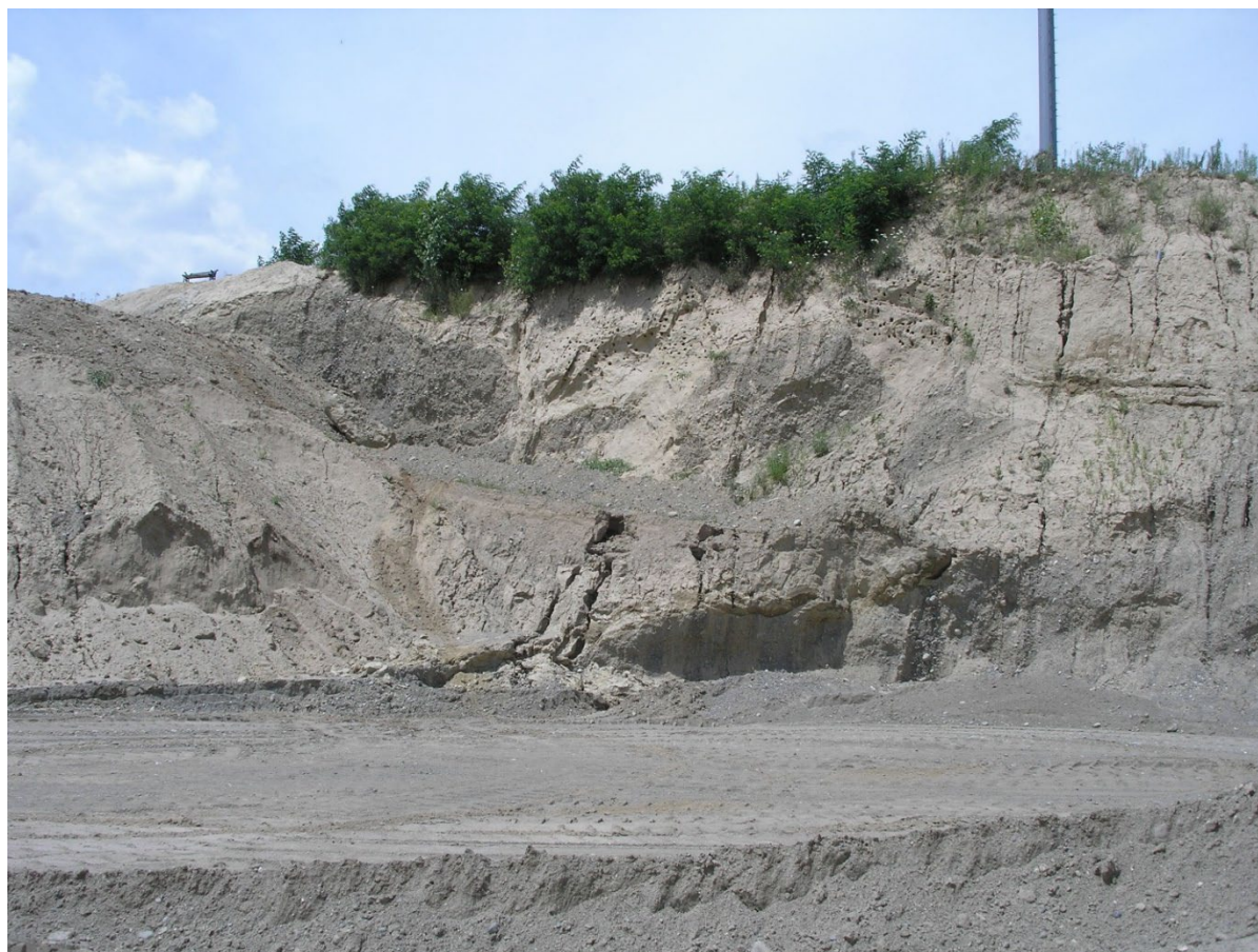
Figure 4.6. Conneaut Sand and Gravel quarry depicting silty sediments contained within a kettle (steeply dipping gravel). Photo by Eric Straffin.
