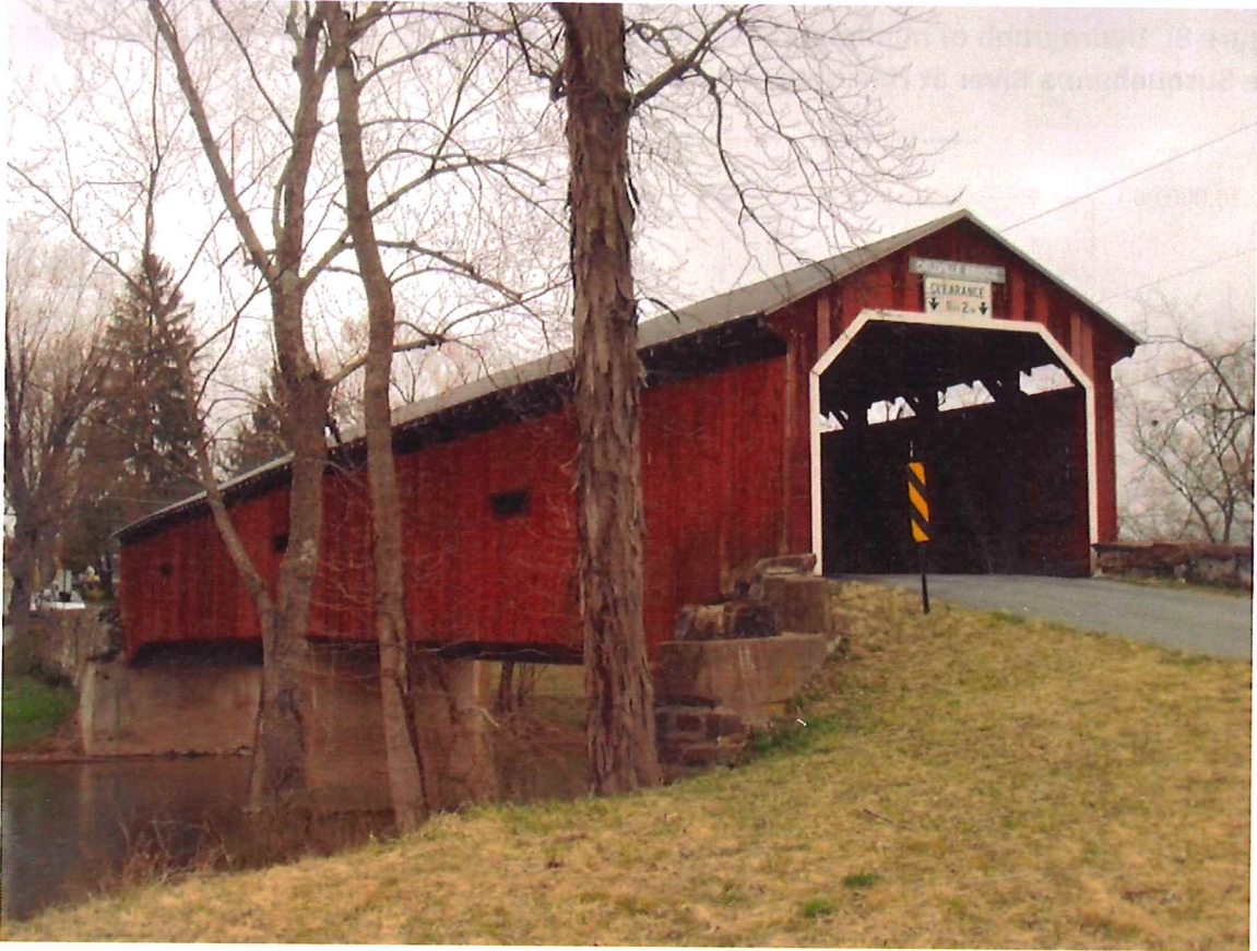
Figure 9: Dellville Bridge over Shermans Creek.
