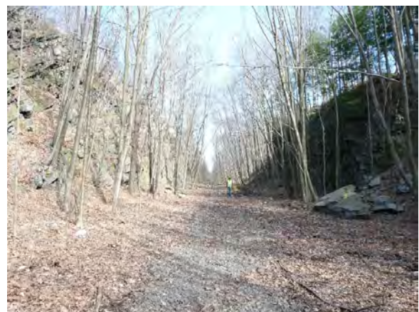
Figure 2. Abandoned Erie Railroad cut through Shawangunk Mountain in the wind gap at Otisville, looking east (GPS 41°28'32.4"N/ 74°33'05.9"W). The cut is 0.15 mi (0.24 km) south of the later tunnel ~100 ft (~30 m) higher in elevation. The beds exposed are northwest-dipping (~30°) quartzitic conglomerate and sandstone of the Shawangunk Formation, the unconformable contact with the Martinsburg Formation being exposed at the east end of the cut (STOP – of this guidebook, p. ----).
