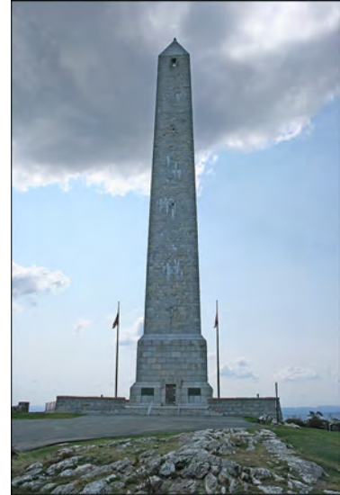
Figure 2. High Point Monument, High Point State Park, NJ.
