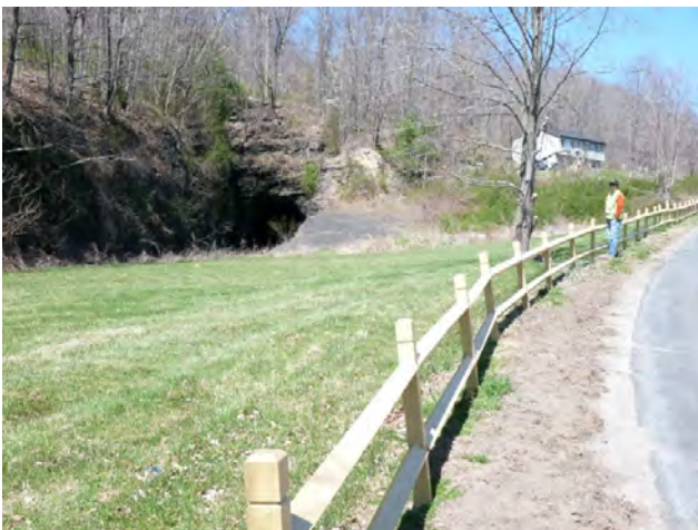
Figure 4. Southeast portal of the abandoned O&W tunnel at High View (GPS ~41°33'30.3"N/-74°27'30.6"W). Bedding in the Martinsburg shale and sandstone in the immediate vicinity of the portal is very gently west dipping.
