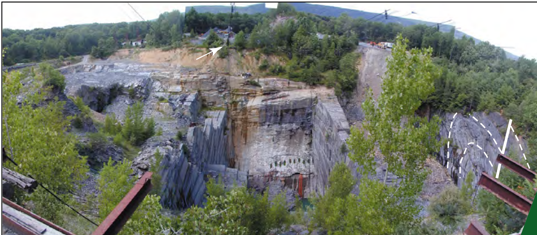
Figure 4. Panorama of quarry looking north. The quarry is divided into four sections: The presently active part is to the left (west). The hole directly ahead is presently water-filled. Two waste-filled abandoned sections are to the far right. A series of oval shapes above the red stain in the central area are 3-ft (0.9-m) wide calyx holes. These are now flooded and no longer visible. The faulted anticline is outlined to the right. The observation point for Figure 3 shown by the arrow.
