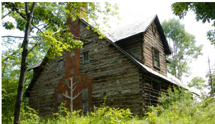
Figure 2. The Outlook Lodge, part of Lusscroft Farm, has some unusual cement artwork along its exterior walls.
