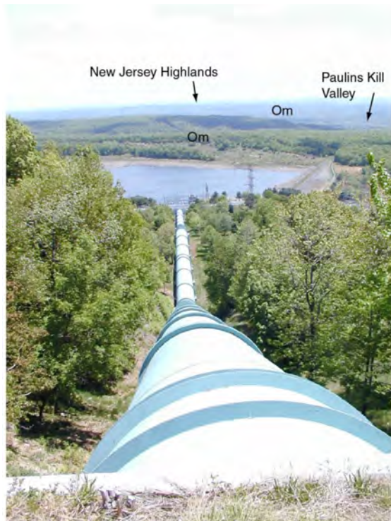
Figure 2. Penstock at Yards Creek from where it enters Kittatinny Mountain just below the Ss/Om contact, to the generating pump plant near the lower reservoir. It is 19 ft (6 m) in diameter, 1,861 ft (567 m) long, and with a 20 percent slope. Three 10-ft (3-m) diameter conduits extend into the plant. Hills of the the Martinsburg Formation (Om) are separated by fault-bounded carbonate rocks of Cambrian and Ordovician age in the Paulins Kill Valley. The New Jersey Highlands, comprising Precambrian rocks are in the distance.
