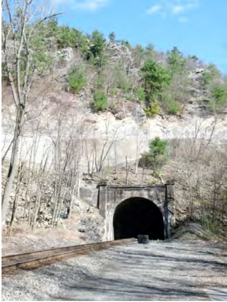
Figure 19. Cliffs of Shawangunk conglomerate at crest of Shawangunk Mountain high above the west portal of the Erie Railroad tunnel at Otisville and just north of the earlier rock cut through the wind gap.
