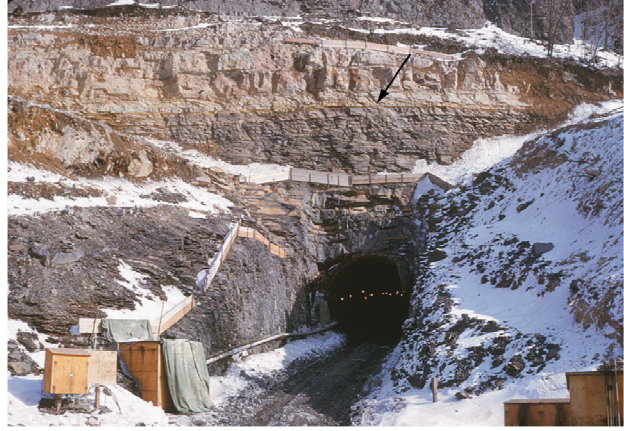
Figure 5. Contact (at arrow) between the dark-colored shale and greywacke of the Martinsburg below the sandstone and conglomerate of the Shawangunk. The slight angular discordance is not noticeable.
