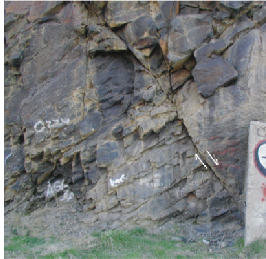
Figure 15. Fault in sandstones and conglomerates of the Shawangunk. Arrows indicate movement directions. The rocks here were coated with soot from trains long departed.
