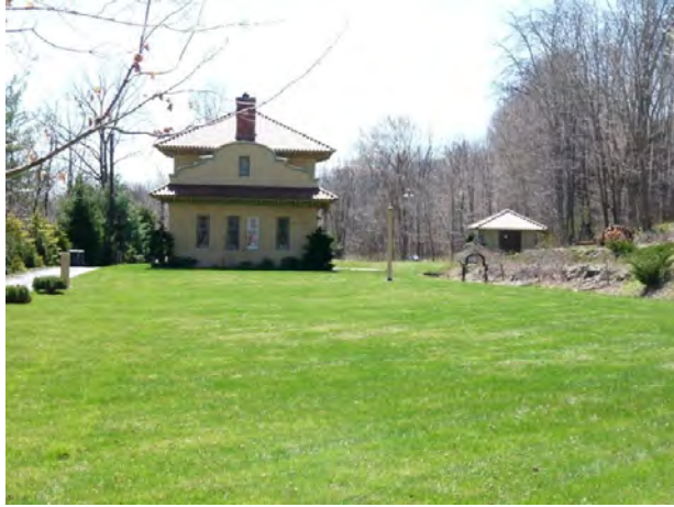
Figure 5. High View Station, now an elegant residence, along the abandoned railroad grade a few hundred feet (scores of meters) from the east portal of the O&W tunnel. In the late 1960's, the station "brood[ed] hauntingly over a field-like thicket, a vandalized shell, nothing more than a shelter for a flock of chickens" (Wakefield, 1970, p. 38). Things have since decidedly improved.
