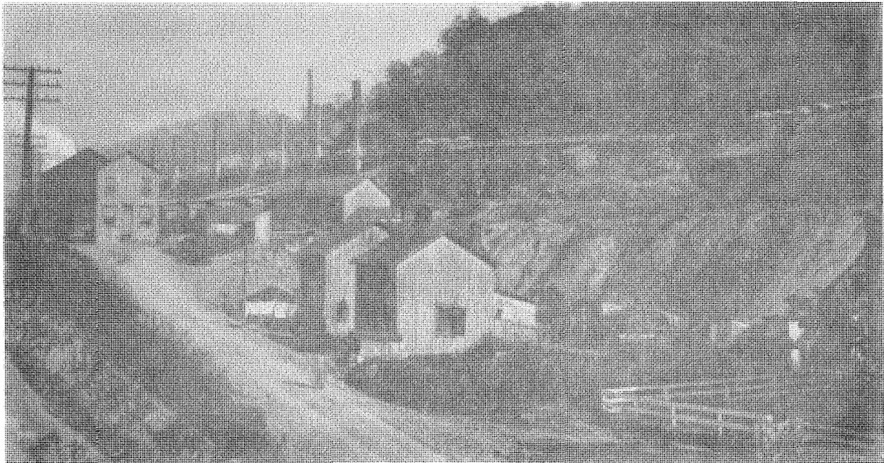
Figure 2. Photograph of 8 vertical-shaft draw kilns at Union Furnace (circa 1916). Railcars of kiln-stone are to the right and on the service trestle or quarry level. Typical quotas for quarry workers were to fill two cars per trick (shift) (Carl Leamer, personal communication, 1986). Wood appears to be the kiln fuel. Northwest face of quarry No. 2 is vaguely visible behind the kiln stacks. Photograph courtesy of Warner Company.
