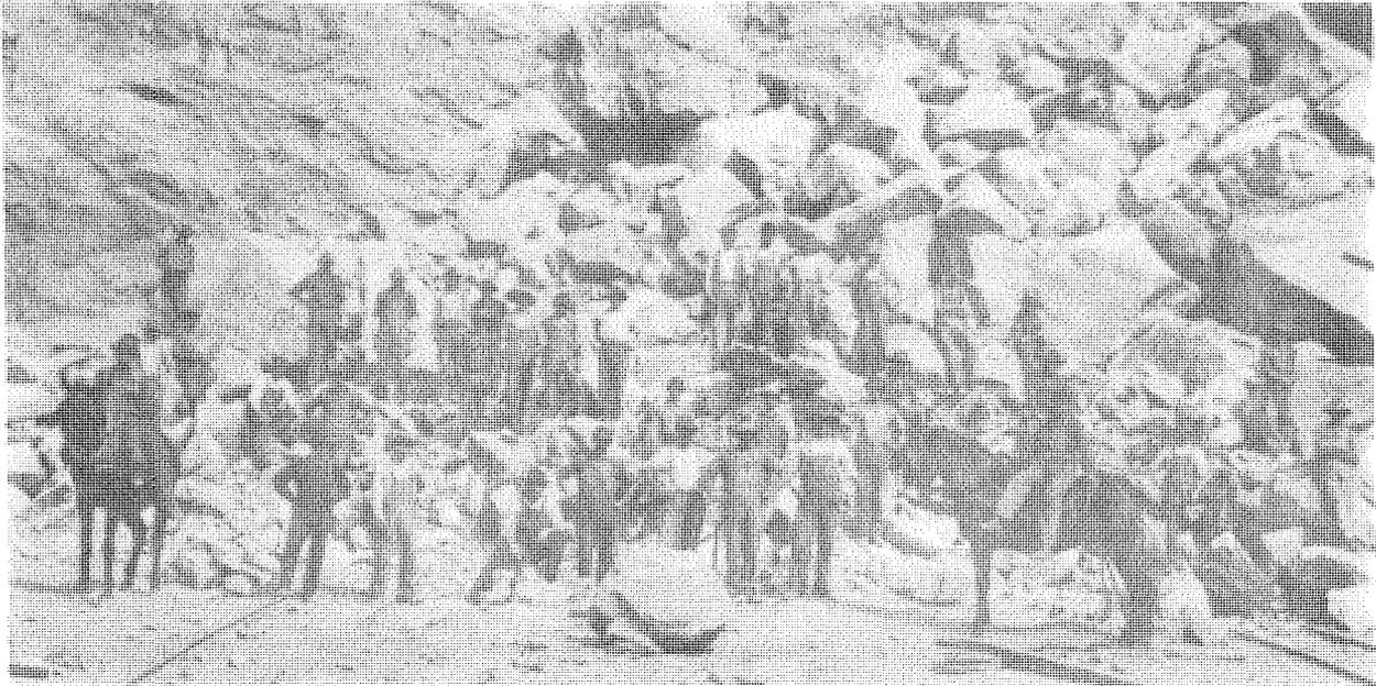
Figure 1. Photograph of Warner Company's Union Furnace No. 2 quarry and work force (circa, 1916). Machine-drilled blast holes are noticeable in the quarry face. Mule-powered railcars apparently transported sized stone from the face to the lime kilns. Notice that pry bars, sledge hammers, and stone forks were required tools in making "little ones out of big ones." Photograph courtesy of Warner Company.
