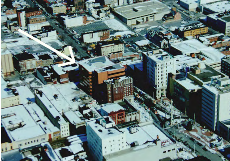
Figure 26. Aerial views of the Corporate Plaza building (arrow) after sinkhole collapse. Hamilton Circle is at the lower right of the photograph.
