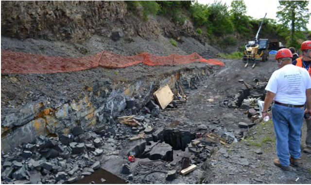
Figure 1-3. Excavation of Finck quarry at Elimспорт by Tera Tek of Salt Lake for static tests of blocks of Marcellus. The excavation parallels the exhumed J1 joint visible to the left. The pit's refuse pile was obtained from this excavation, now filled. Photo by Terry Engelder, PSU.
