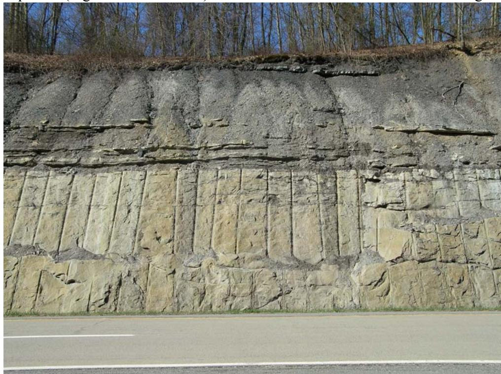
Figure 12-9. Thick middle sandstone at STOP 12 exposed in canyon-like exit ramp of Toll 60 North. Bedding planes and primary structures are very difficult to see. Subtle discontinuous horizontal fractures are planar bedding planes.
