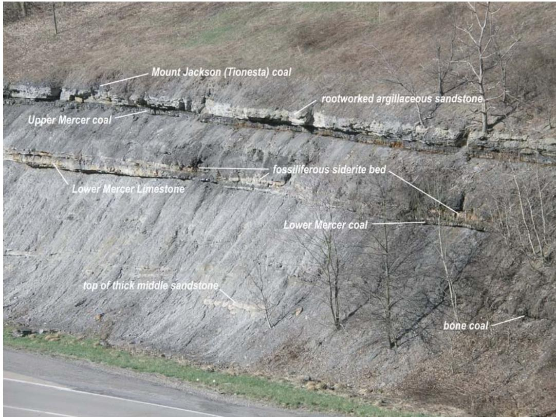
Figure 12-12. Termination of Lower Mercer Limestone exposed along eastbound US 422 near entrance ramp of Toll 60 South. Fossiliferous siderite bed continues throughout site. Upper Mercer coal is only three to four feet below Mount Jackson (Tionesta) coal here, separated by rootworked argillaceous sandstone.
