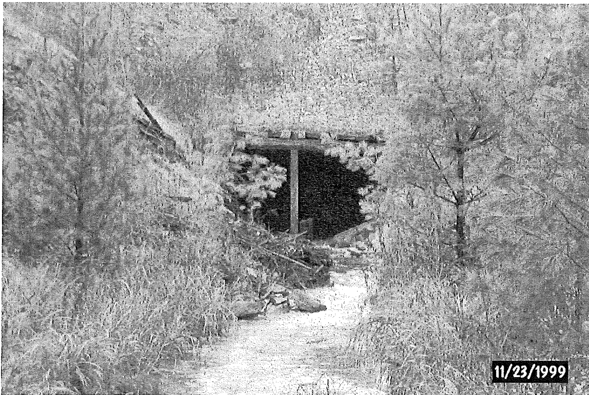
Rowe Tunnel Discharge.
